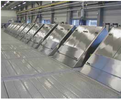
Meva Monoscreen in a WWTP
