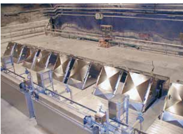
Meva Rotoscreen in a WWTP
